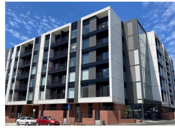
Hauwai Apartments is an impressive building, being a new-build structure providing 93 completed apartments. The site required robust ground-work including new inground services infrastructure to King Street and Adelaide Road, and circa 160x 12-15m deep concrete piles. The structure is a hybrid precast panel and in-situ concrete solution, including the floor slabs which are supported on a precast rib and infill system. The resulting structure provides solid concrete inter-tenancy walls.
